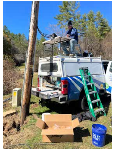
These damaged cables were too short to reach the ground and had to be repaired from a truck's roof.
